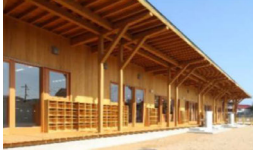
Medium-sized and large wooden structures – metal-joints method
