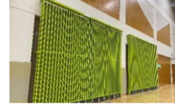
Dehumidification-type radiator heating and cooling system
