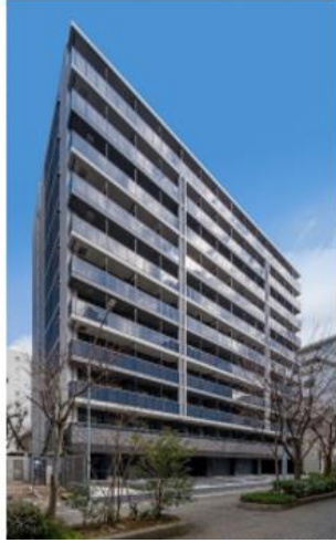
Exterior of building's southwest side
